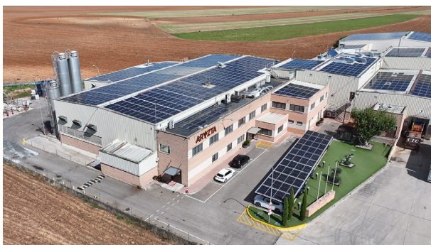
Figure 4: Solar Panels across our Madrid Bakery
